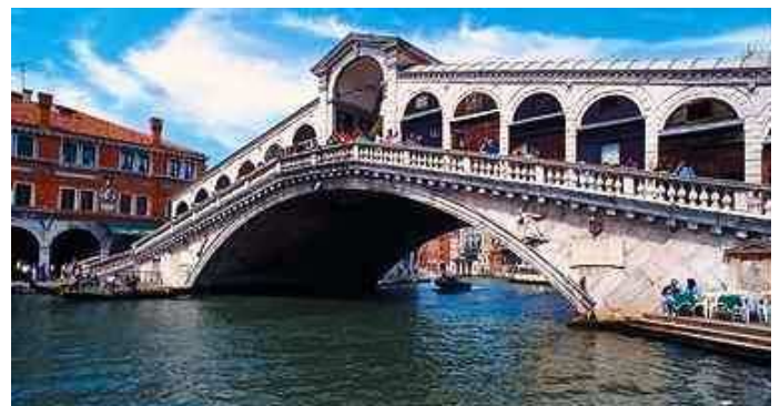
Rialto Bridge in Venice, Italy.
